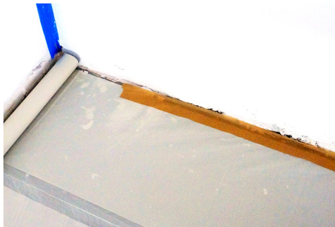
Don't forget to protect the ground with a protection tarpaulin.
