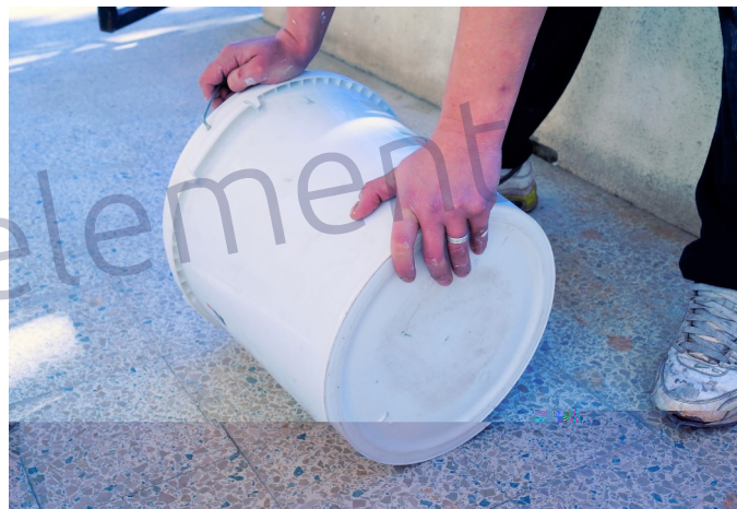
Roll the bucket of waxed concrete before opening it to decompact it.
