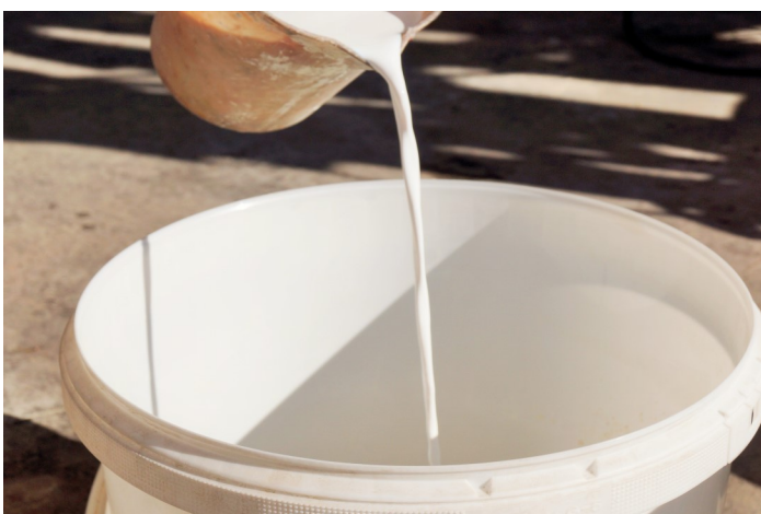
After measuring the quantity of resin required, pour it first into an empty bucket, then add the powder.
