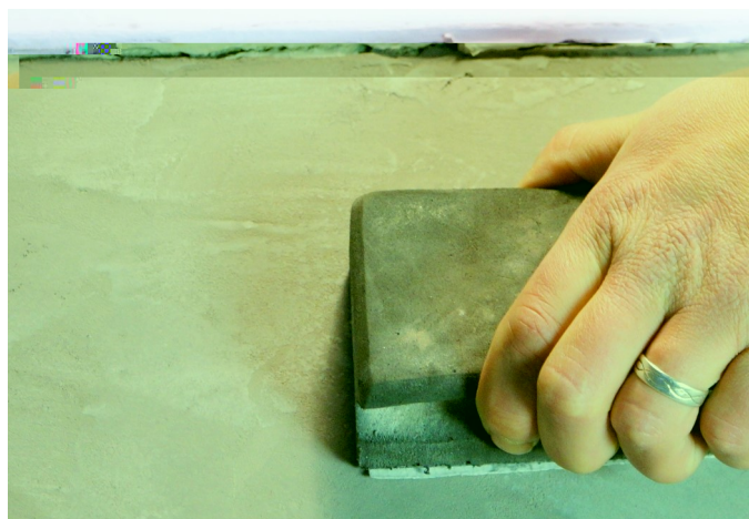
To facilitate sanding at the edges or corners, use the sanding block.
