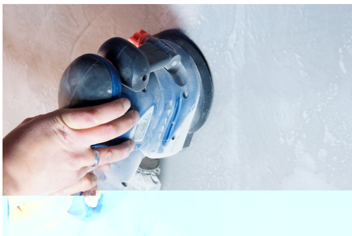
24 hours after the application of the second layer of waxed concrete, sand the surface with a disc of 80 then 120.
