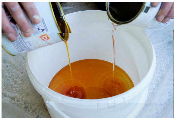
Pour the 2 components A and B in a clean bucket.
