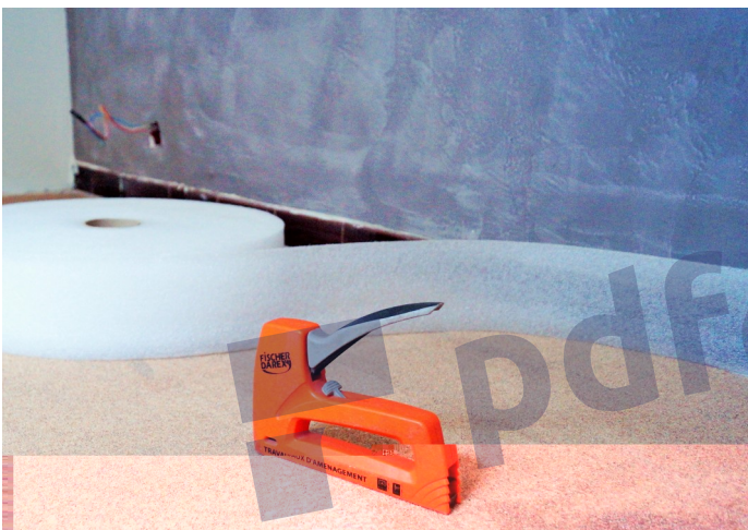
The peripheral strip allows to protect the walls and to separate the wall from the ground.
