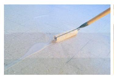
Depending on the type of surface, apply the Prim or Prim plus either with a 250 mm roll or with a 500 mm roll.
