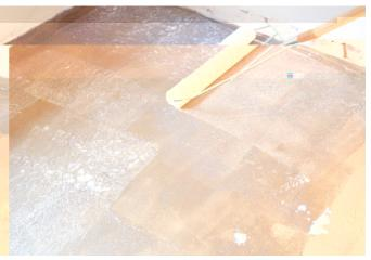
On a closed surface, apply the Prim or Prim plus either with a 250 mm roll or with a 500 mm roll.
